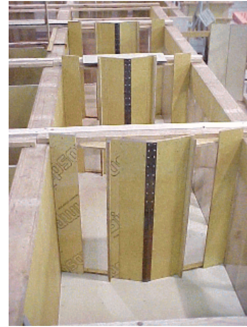
View of chevron shaped dual-vertical slot baffle fishway looking downstream.
